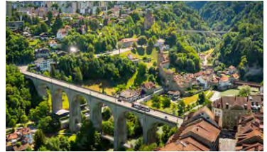
Pont de Zaehringen Zähringerbrücke Zaehringen Bridge (1924)
